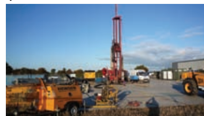
Drilling at Fradley Junction ▼
