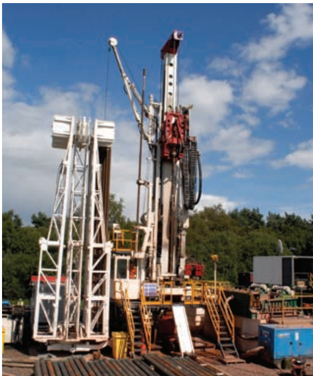
< Drilling at Willoughbridge in Pedl 78
