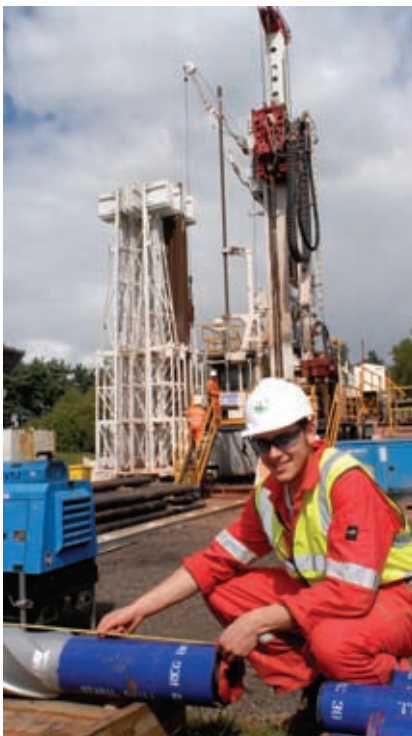
< Drilling operations in Staffordshire
