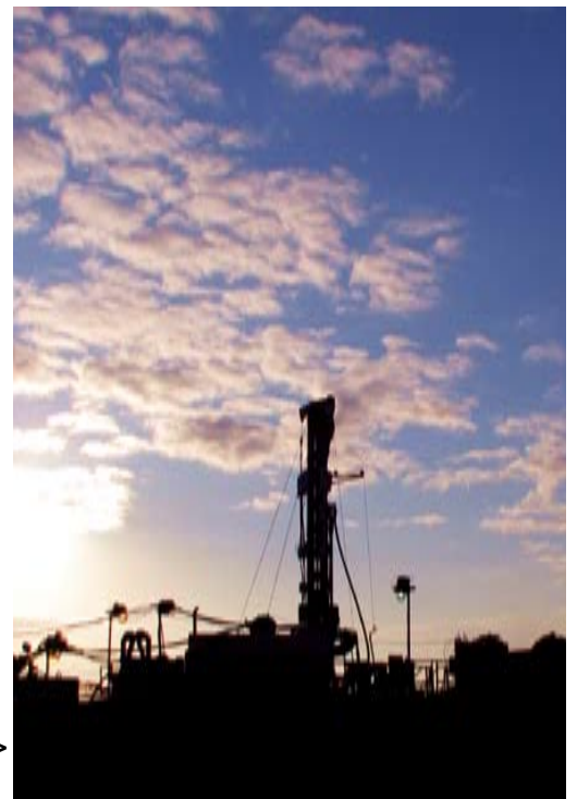
> Drilling an assay well Fox Hill Farm on the outskirts of Liverpool. This well was logged and cored in April 2008
