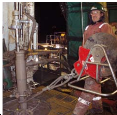
Drilling activity at Doe Green >
