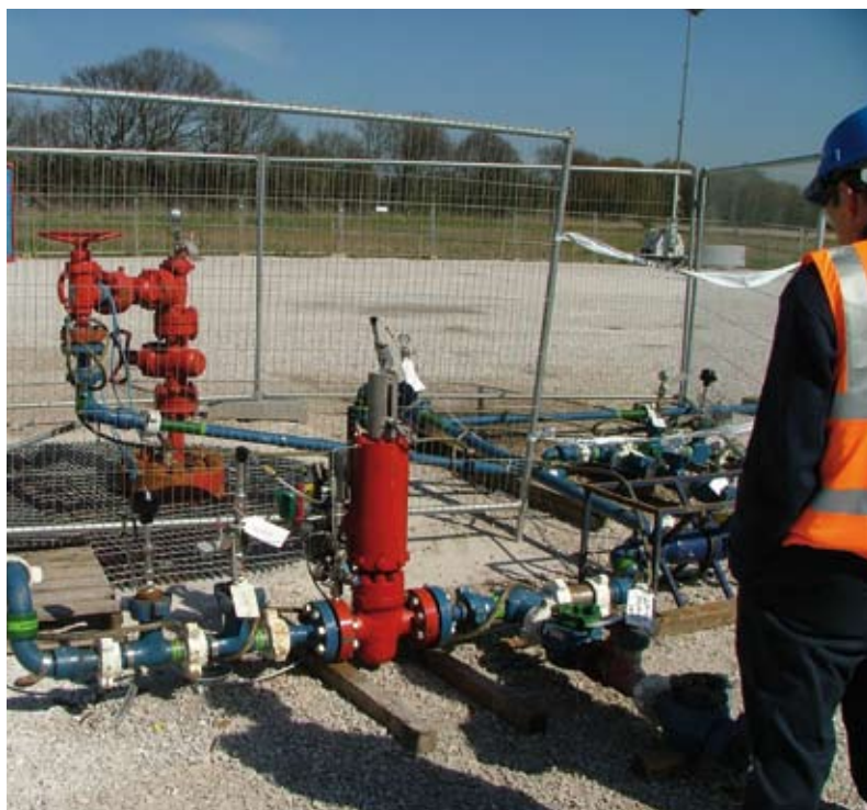
< Monitoring the production test at Doe Green
