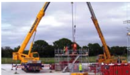
^ Working over a well at Doe Green using cranes
